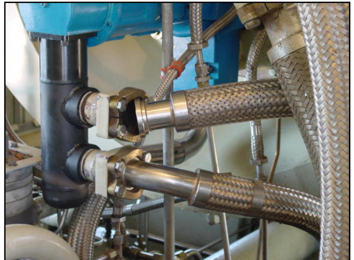
Figure 8. Exhaust Hose Installation
